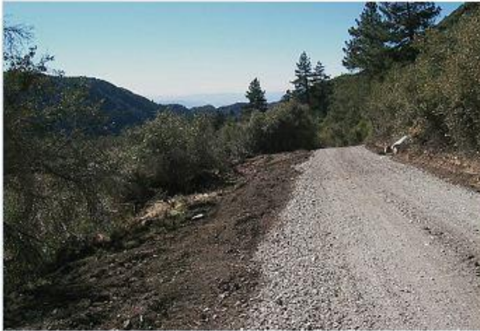
Figure 32: Example of an outside sloped road (Photo R. Harris in Kocher et al., 2007).
